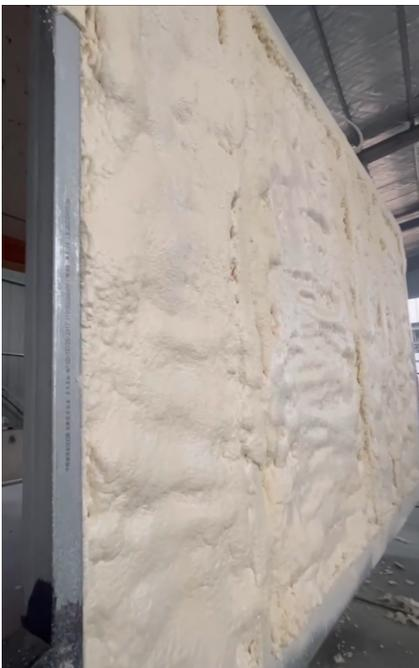
Insulation R ratings\* A 150mm thick polyurethane foam insulation layer will typically have an R-value between R-22.5 and R-42, depending on the specific type of polyurethane foam.
